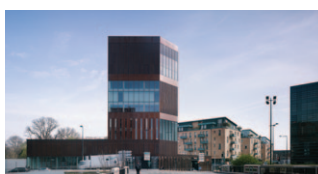
TOUR EURAVENIR LAN - Local Architecture Network Lille (59) - 2014 - © J. Lanoo
